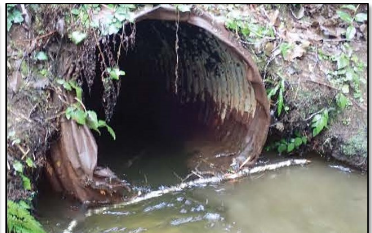
Rover Creek Culvert Replacement Project Adriana Morales, SNF Hebo Ranger District
